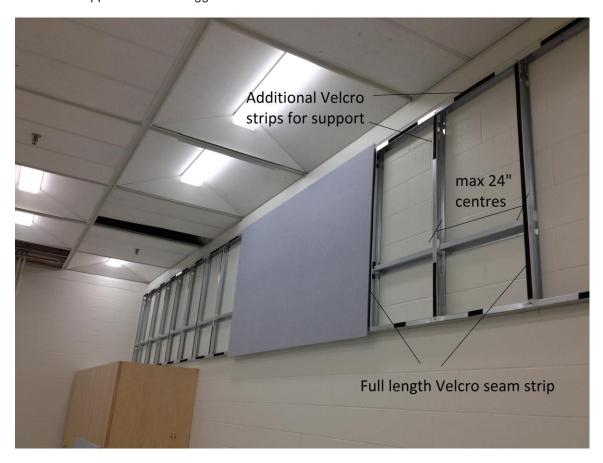
The contractor has applied single full length Velcro **self adhesive** strips on the centre of the studs where the seams of 2 adjacent ezoBord panels will meet. This is important for tight seam alignment. Shorter strips have been placed in other locations on the framing for additional panel support.
